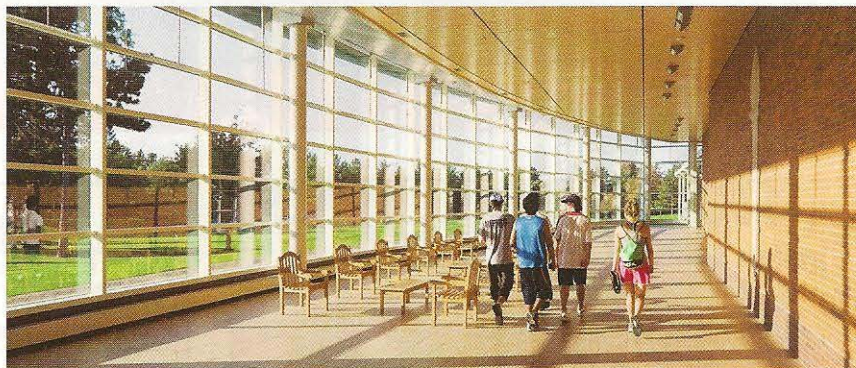
The glass-curtainwalled entry lobbies wrap the larger-volume brick "boxes" housing the activity space.
