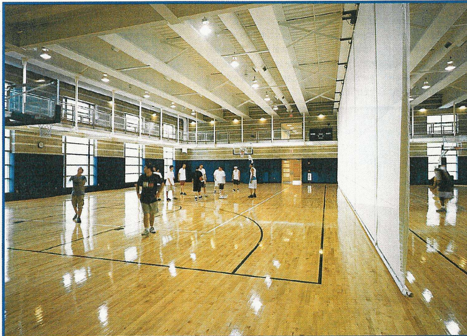
Long-span structural demands dictated that two gyms be stacked at the facility's uppermost floors.
